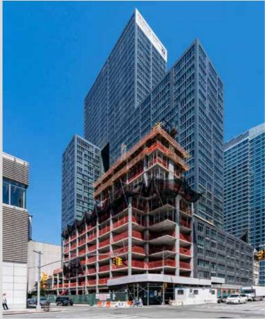
in this project. The RKS platforms were pre-assembled and delivered to the jobsite. Finally, for the shoring construction, the client used ULMA's CC-4 Aluminium Modular Formwork , which provides excellent concrete finish, and it is perfect for solid or lightened slabs.
